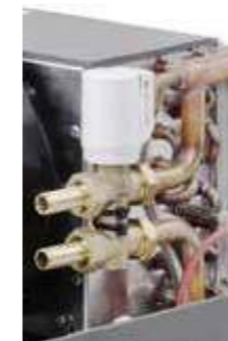
Electric heating element and three-way valve
